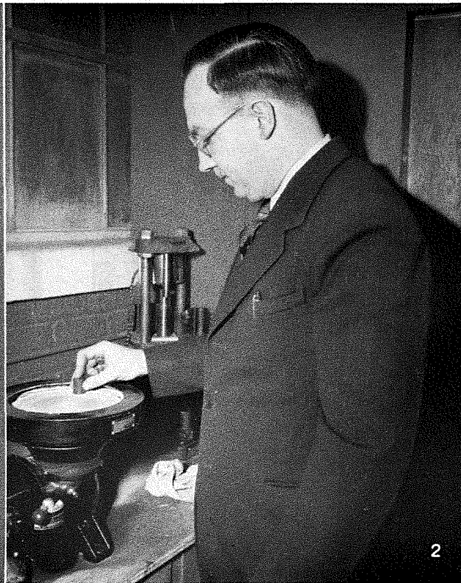
2. The section of metal is polished, first with decreasingly smaller sizes of emery paper, then with a wheel and fine emery powder.
